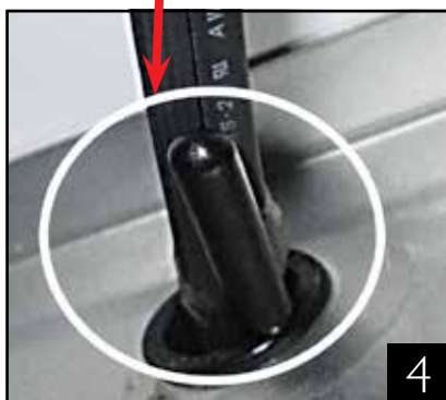
Close-up of black probe next to power wire at bushing.
